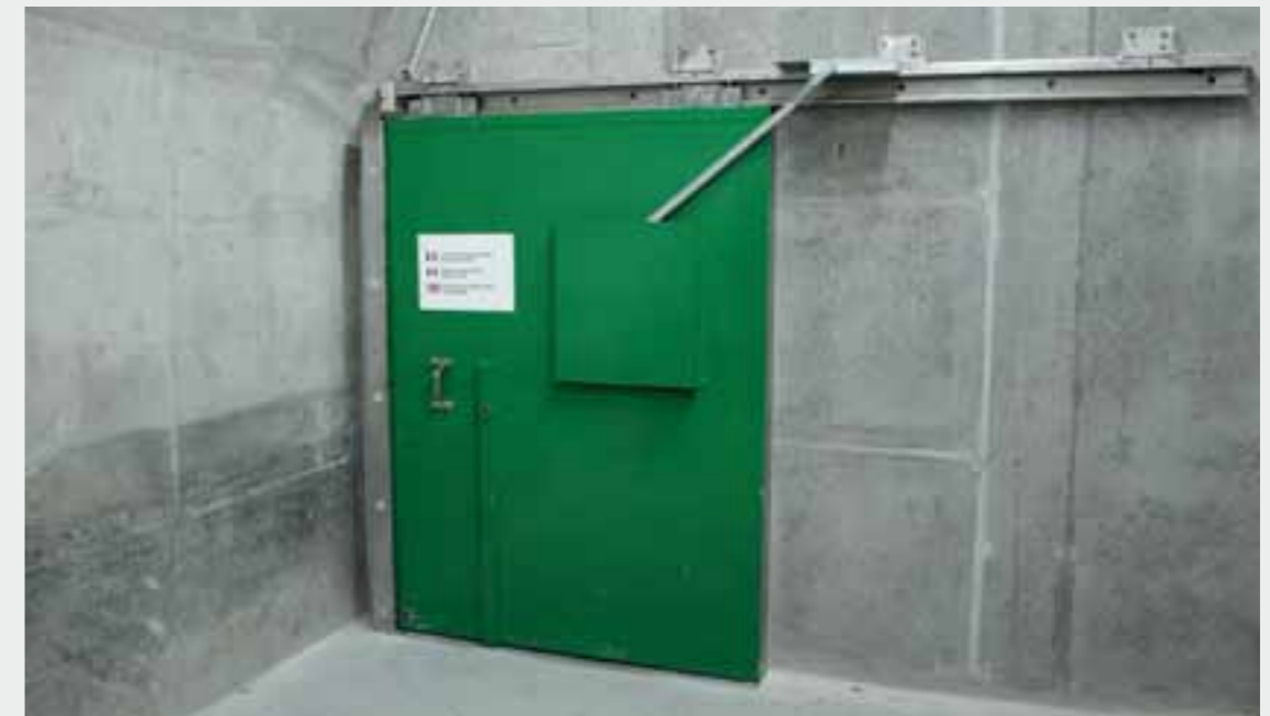
Tunnel Fréjus, Frankreich|Tunnel Fréjus, France|Tunnel du Fréjus, France|Túnel Fréjus, Francia
