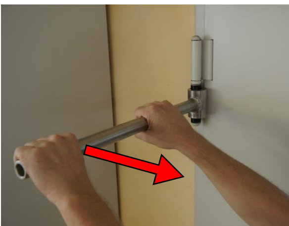
Figure 3: Bend the lower part of the hinge inward
