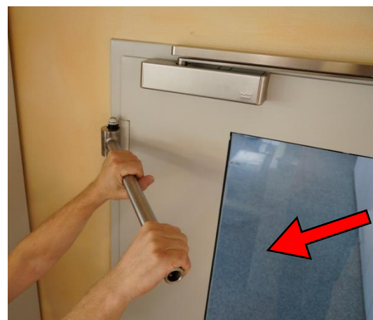
Figure 4: Bend the upper part of the hinge outward
