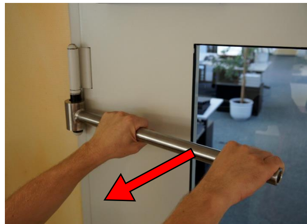
Figure 2: Bend the lower part of the hinge outward
